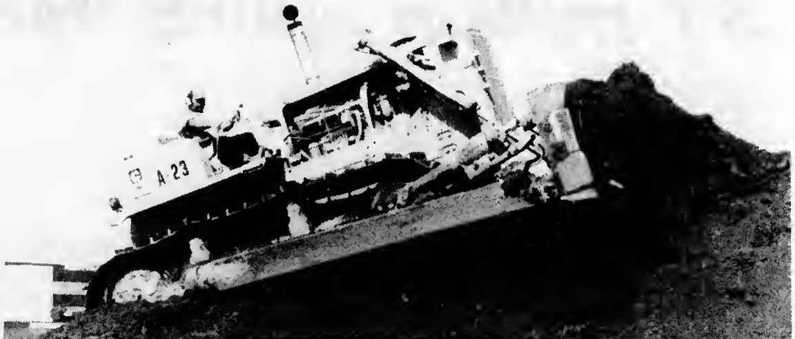
Expensive dirt —as construction costs will total about $67,000 for the White extension lot. The lot is expected to be ready by November. Photo by Trilby Bittle.
