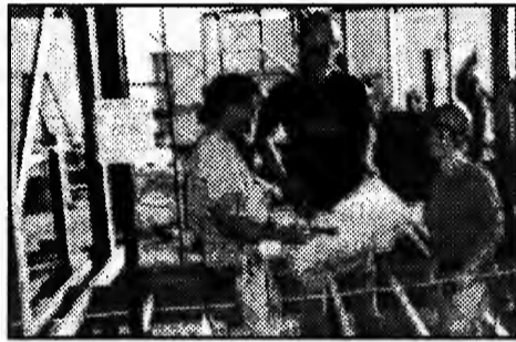
Progress in work.. construction continues in the concourse.
