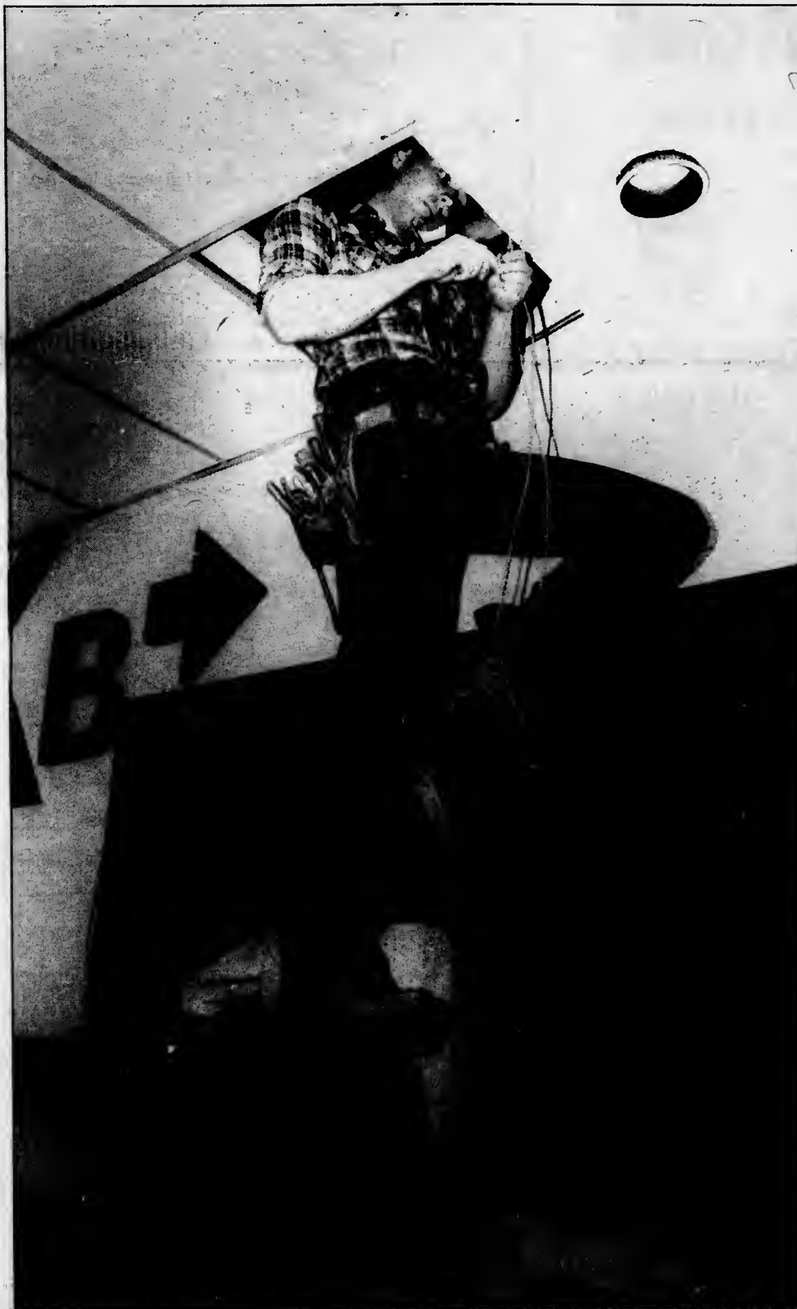
Wire you insulate? —Pay telephones at Humber were more than out of order last week—they were out of the building. Bell Telephone installer Braden Baron prepared the wiring for installation of new telephones, in the lower level near the Pipe. (See page two for another photo.)
