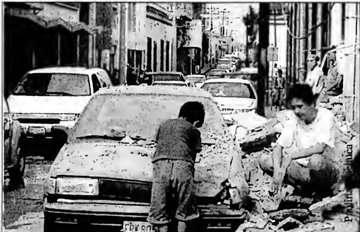
Vehicles damaged from falling debris from surrounding buildings and offices in downtown Colima.
