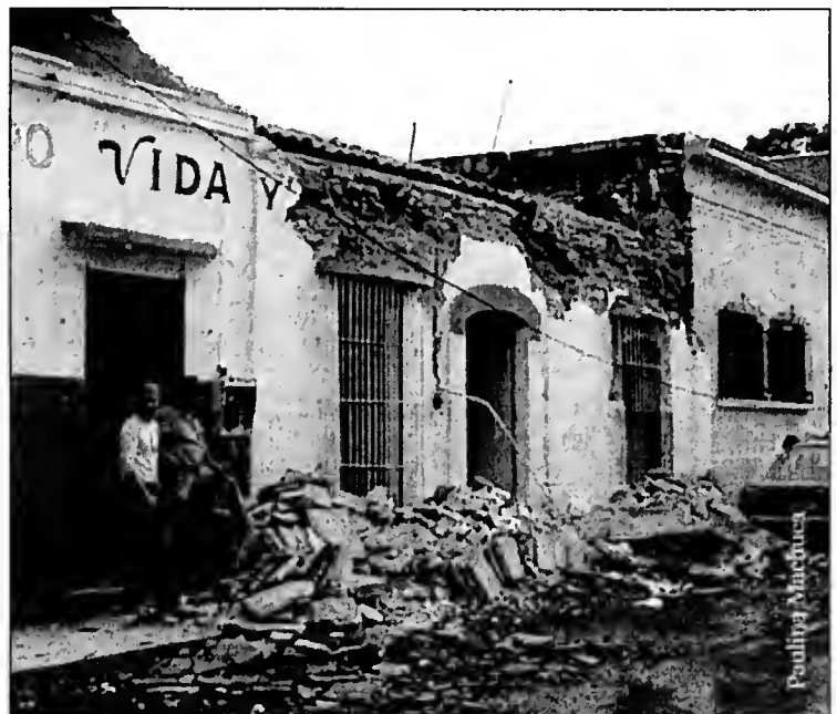
Fragile adobe houses easily damaged in Colima, Mexico where the earthquake hit the hardest. Residents moved into nearby town of Tecoman due to threatening tidal waves.
