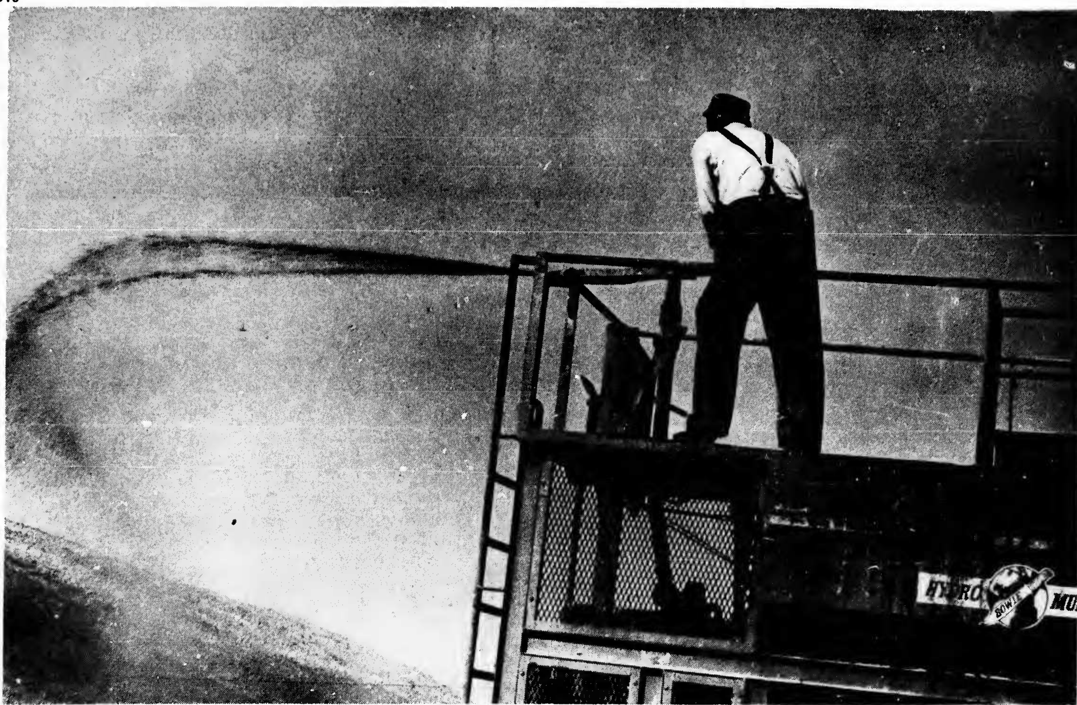
One can't help but notice Humber's idle ski hill is now green. The green conglomerate of peat moss, seed, fertilizer and a chemical hardener is called 'Instant Sod', applied to the hillside by a high pressure gun. While Jack Frost changes the green leaves to brown, Humber College changes the brown hills to green.
