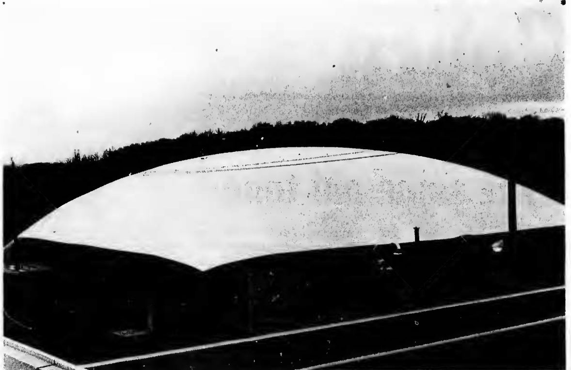
It's up again. After two weeks of renovations, the new translucent bladder will provide better lighting by allowing outside light in and reflecting inner light properly. Also, an improved means of holding the covering down using 700-lb. cement blocks will lessen the work involved in taking down and putting up the Bubble.
