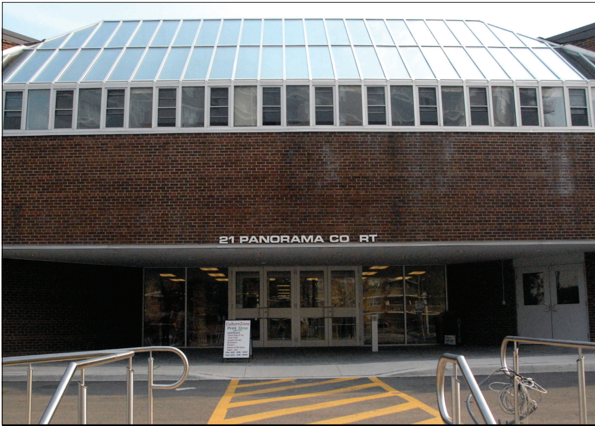
PHOTO BY ALEX KOZUSZKO What was once Father Henry Carr Middle School is now home to 11 agencies that offer a wide range of social services to the entire Rexdale community. Its creation resulted from a United Way report on priority districts.
