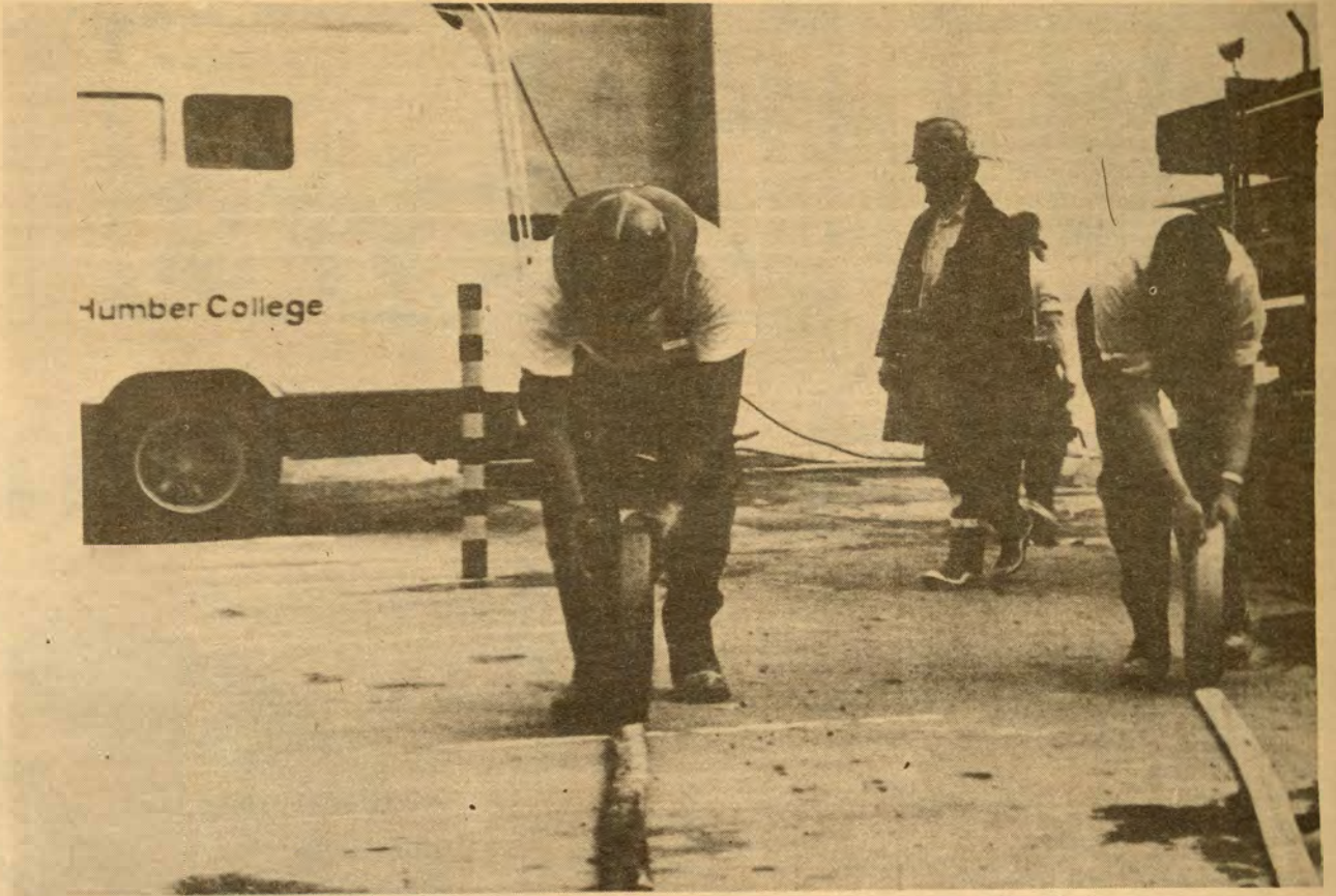
After battling the quarter of a million dollar blaze the job of cleaning up had to be attended to.
