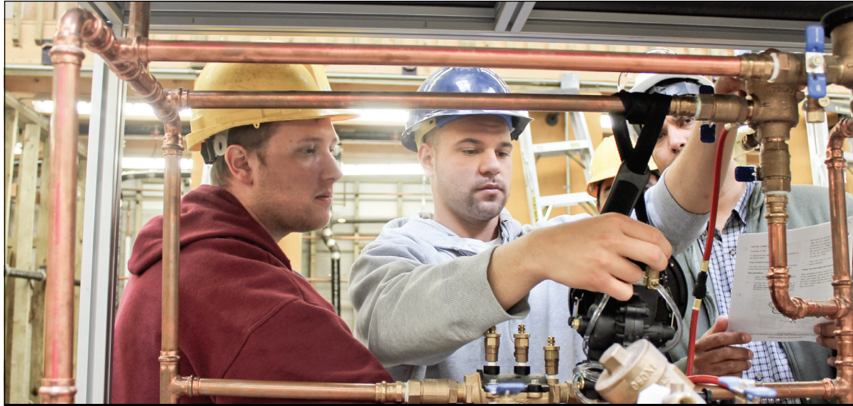
PHOTO BY KRISTIN ANDREWS Humber plumbing apprentices (from left) Arthur Chamie, Robert Butera and Ashad Mahmood.
