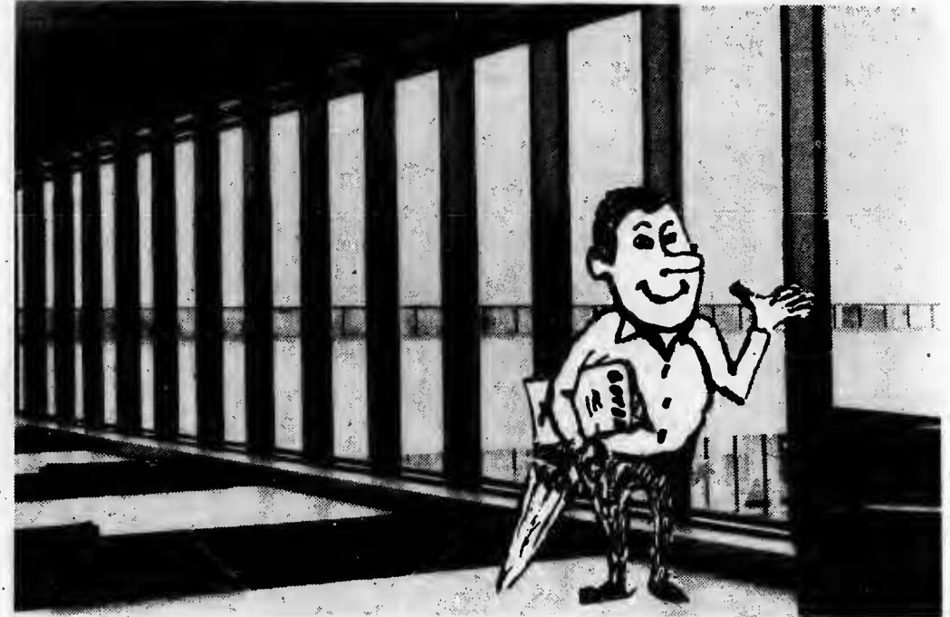
Leaking library window baffles college. Photo by Borys Lenko.
