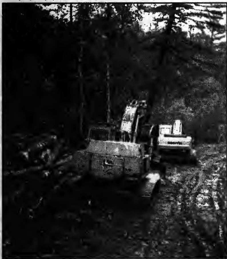
ABOVE: Lea Ann Mallett shows Earthroots members the full-page ad that Now magazine published for free. BELOW: Goulard Lumber Company's equipment sits dormant due to heavy rains last Friday.
