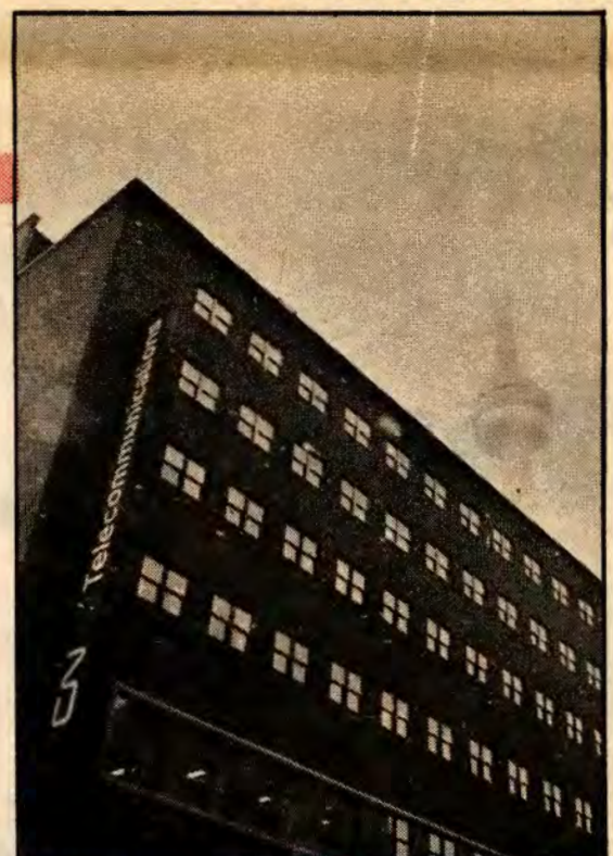
Tracking of the tower will be done by CN telecommunications.
