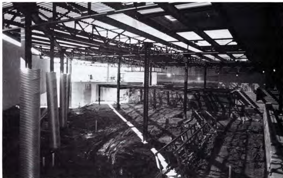
The new Student Centre under construction
