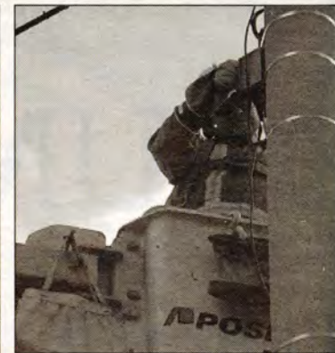
Toronto Hydro workers fix the crosswalk near North Campus.
