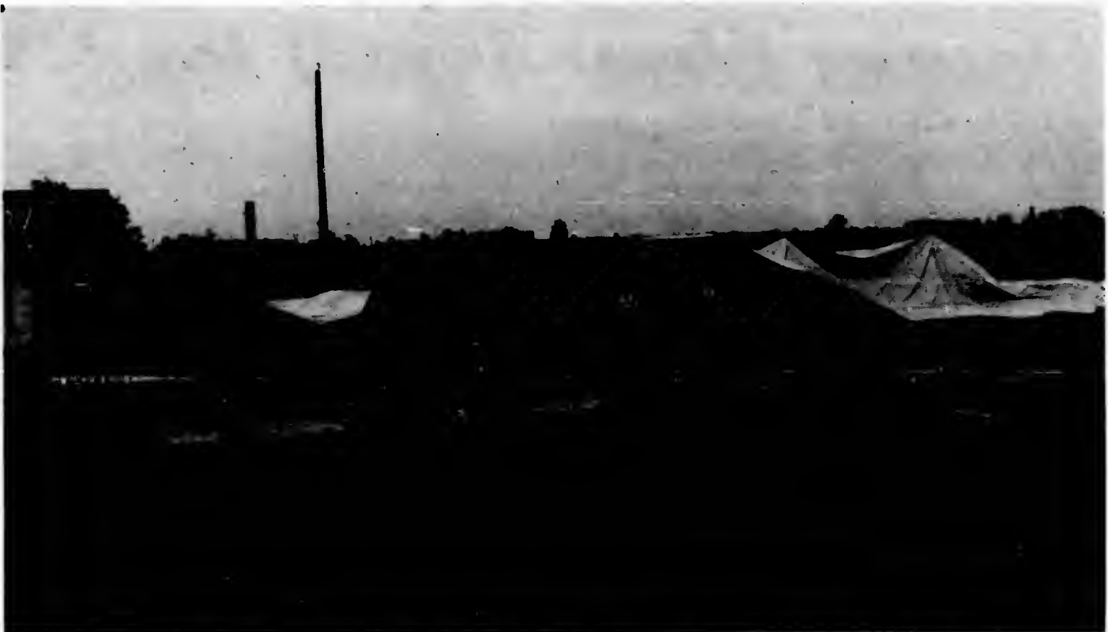
Pop goes the Bubble: Humber's deflatable gymnasium had its air let out Hatton, athletics co-ordinator for the Centre for Continuous Learning last Thursday. Structural repairs will have to be made, and Michael says it should be up by this week. (Photo by Steve Wilson)
