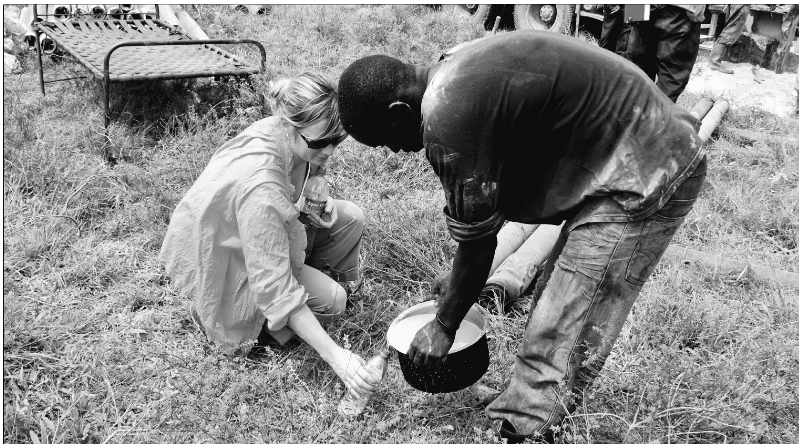
Interior design program co-ordinator Kelly Gluck at the building site in Lyantonde, a small town in southern Uganda.
