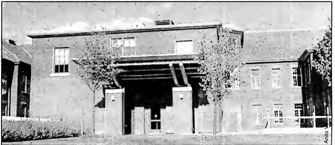
A renovated Building F now houses the Media Studies program which moved to Lakeshore from the North campus this year.
