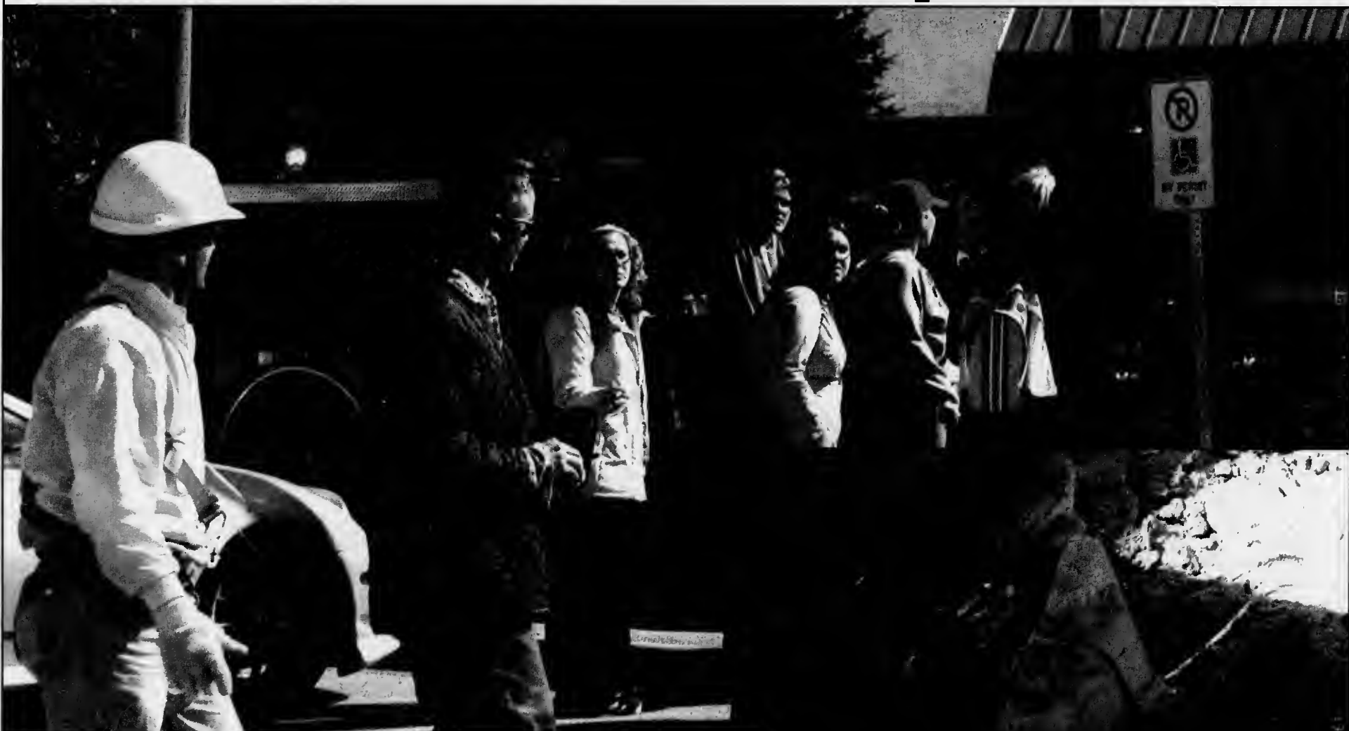
Emergency staff evacuated both rez buildings and construction crews at the new residence site Tuesday morning after workers from Four Winds Construction Inc. ruptured a gas line with a backhoe near the residence loading dock. Enbridge Gas capped the line and gave the all-clear after an hour and a half.
