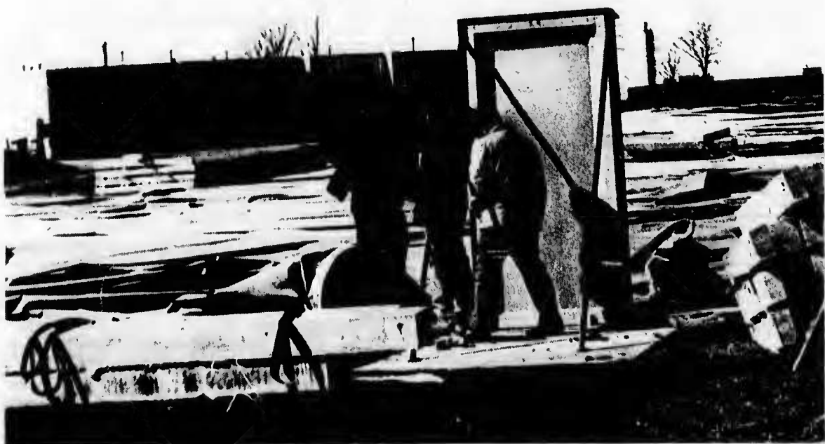
A door that leads to nowhere. It should lead to the Bubble, but it was taken down for repairs on Tuesday morning. The skin is going to be replaced by one with a white ceiling, so that the light will be reflected better. It should be up by the weekend.
